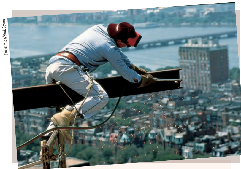
Build with care The chance of a construction worker being injured at work during the year is 1 in 27.
